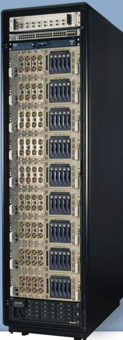
▲ Microway® Quad Optron™ Cluster with 36 Optron 880s, redundant power, 45 hard drives and Myrinet™ in our CoolRak™ cabinet.
